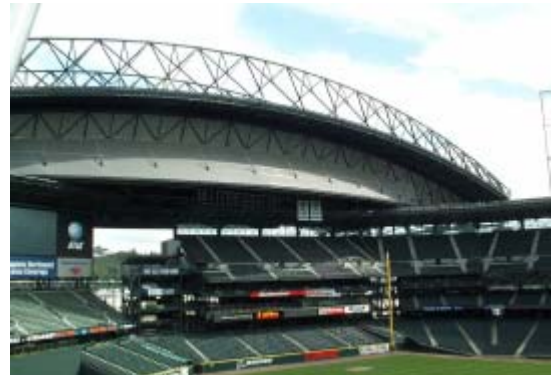
A view from inside SAFECO Field with panels fully open
