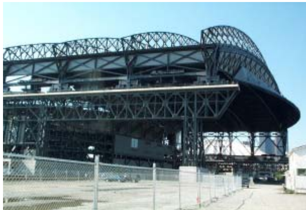
A view of the panels from the outside of SAFECO Field
